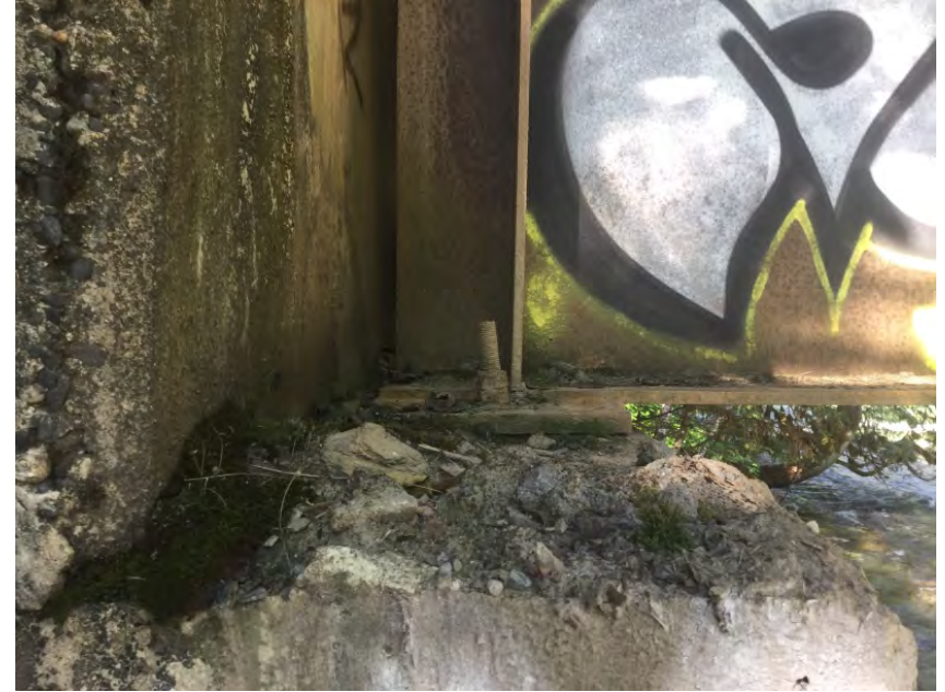
Upstream left bearing bolt
