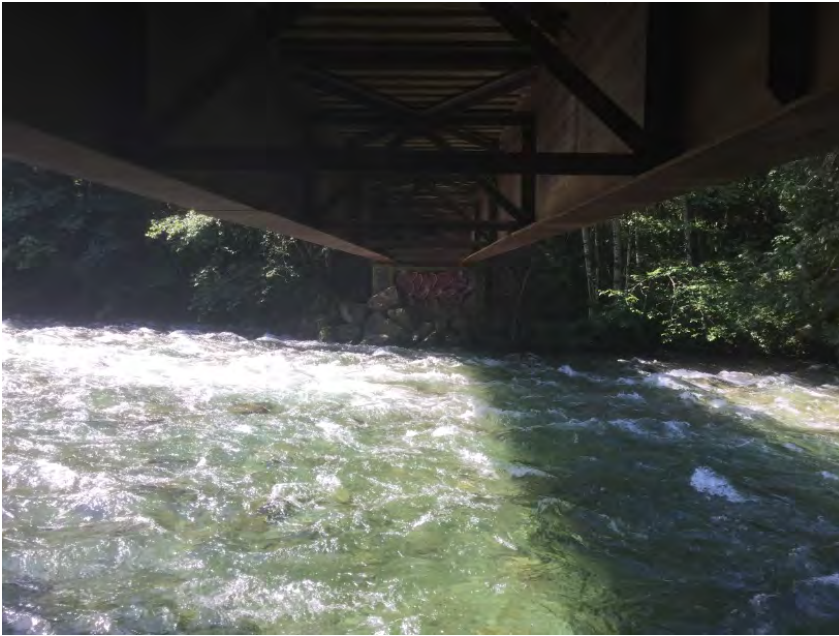
Left Bank Abutment when facing downstream
