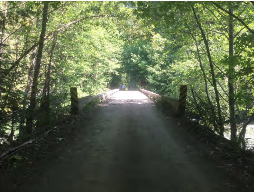
Approach from Left Bank when facing downstream
