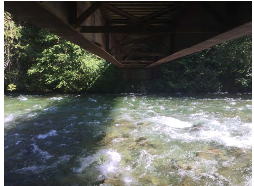
Right Bank Abutment when facing downstream
